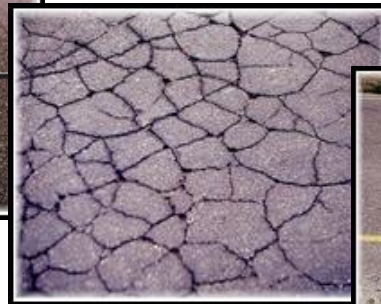
Fatigue Cracking
